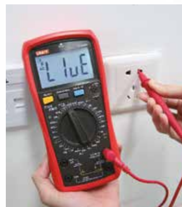
Live and nature wires identification
