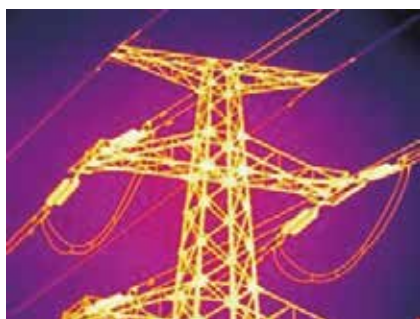
Power line inspection
